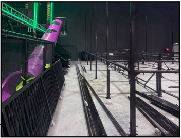
Netting Columns: 60×60×3 (mm) square tube + softwrapped column
