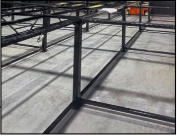
Main Columns: Square tube 90×90×4 (mm)
