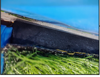
18mm plywood + 4cm EVA + artificial turf
